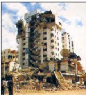
Fig. 3.3a: Destruction caused by an Earthquake in Gujarat
