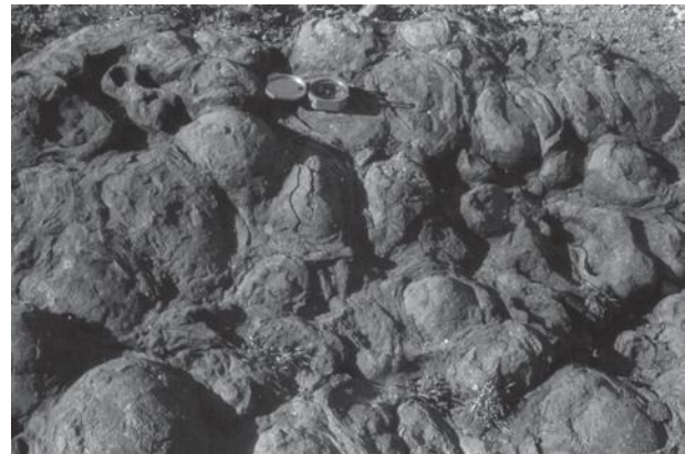
Fig.6.4 : Exfoliation (Flacking) and granular disintegration
