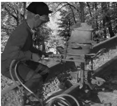
Figure 3.11 Thermit process for joining railway tracks
