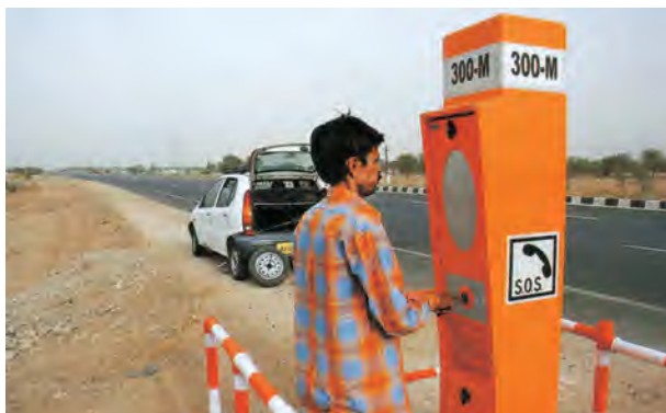
Fig.7.10 : Emergency call box on NH-8
